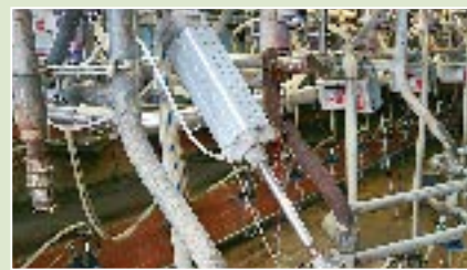
Gates that draw on vacuum supply are bad news; they cause vacuum fluctuation. Upgrade to a compressed air system, as the ram can usually be adapted to cope.
