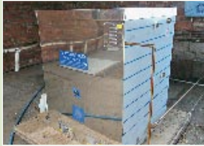
Upgrades should also include a look at the hot water system. Modern systems use heat from the incoming milk to reduce heating bills. Having sufficient hot water volume is also important bearing in mind the larger diameter pipes that need to be cleaned.
