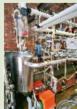
Vacuum lines should be looped back to the header tank; this has a positive effect on milking efficiency. Large-diameter piping creates a vacuum reservoir.
